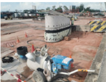
Thomson Line MRT Project Singapore
