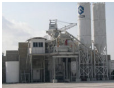
Syscon Pte Ltd, Singapore Precast Factory
