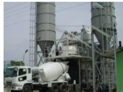
Sunpower System Pvt Ltd, Sri Lanka Water Treatment Plant Project
