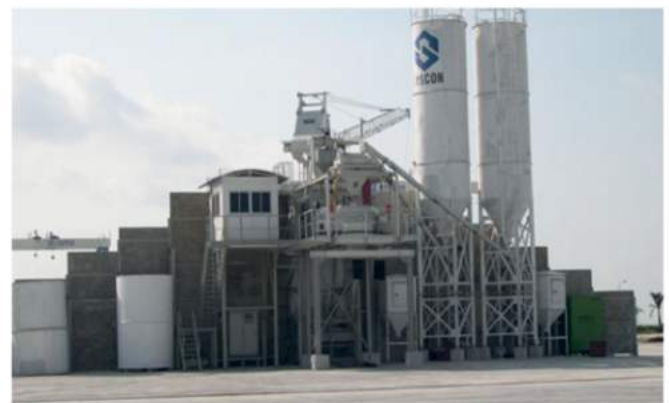
Syscon Pte Ltd Precast Factory SINGAPORE
