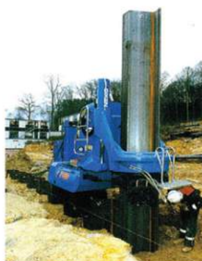
Silent Piling Machines
