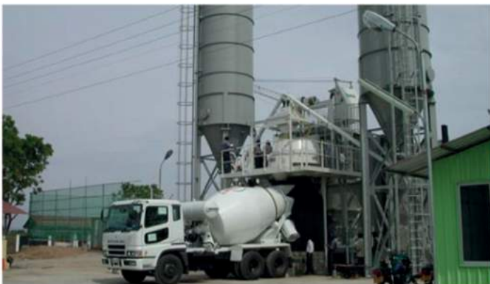
Sunpower System (Private) Ltd Water Treatment Plant Project SRI LANKA
