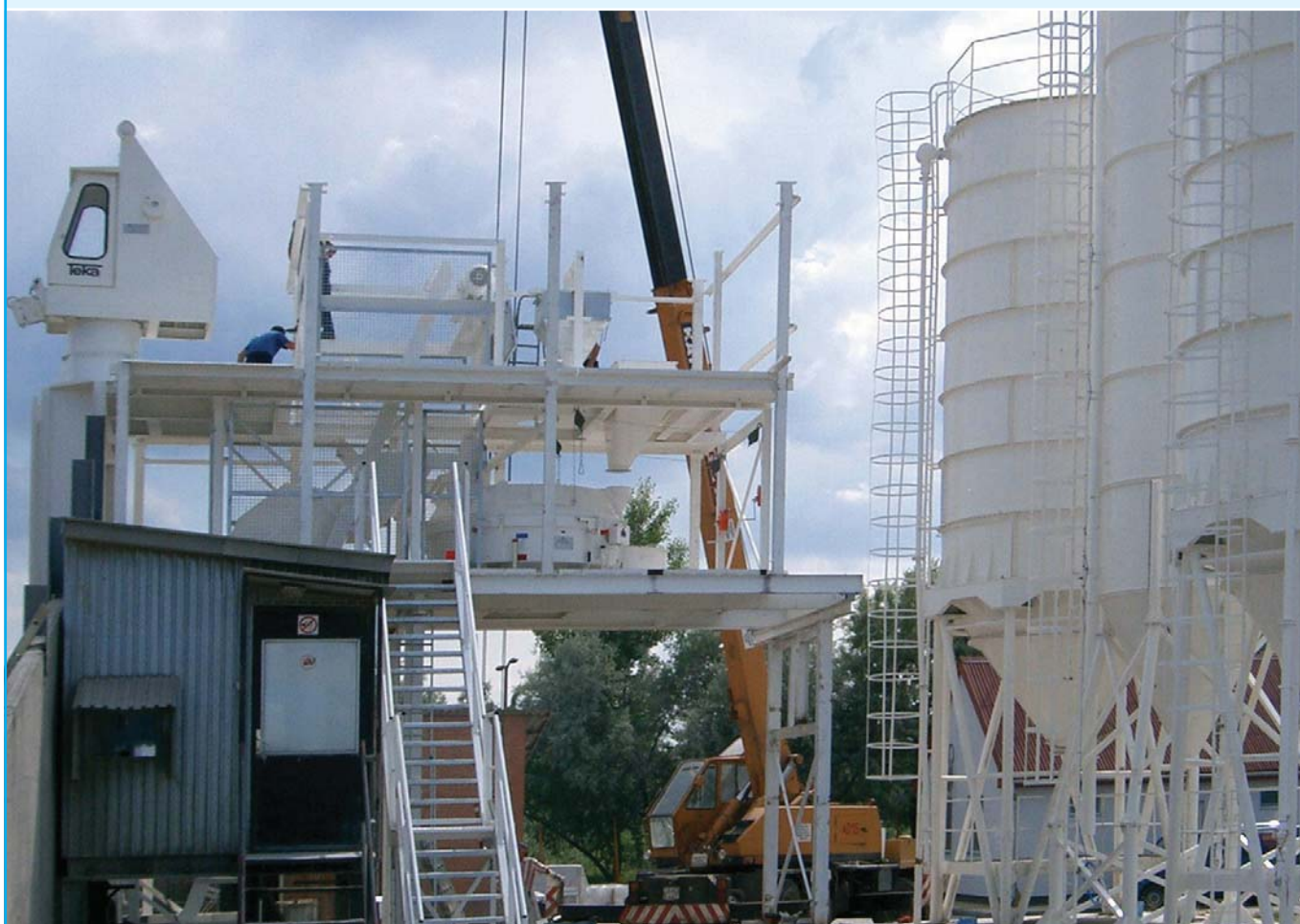
Montage MIXOMAT THZ 1500 B - S 5 Sternanlage • Erection MIXOMAT THZ 1500 B - S 5 scraper system
