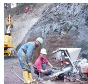
Injection of self-drilling anchors
