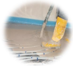
Self Levelling Floor Screed
